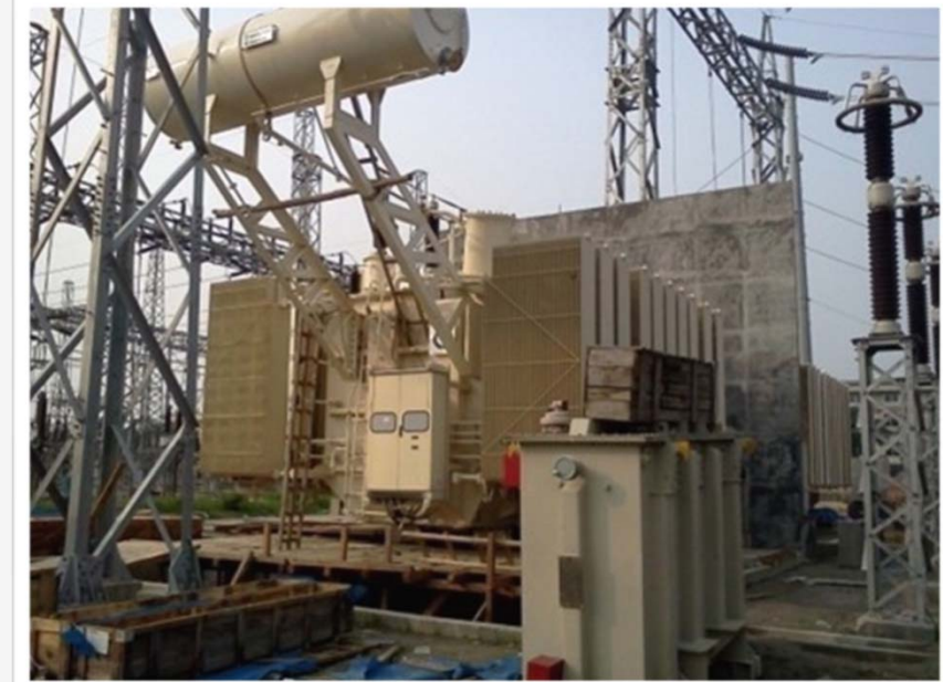
Fabrication of 230kV Transformer(Nov.09, 2012)
